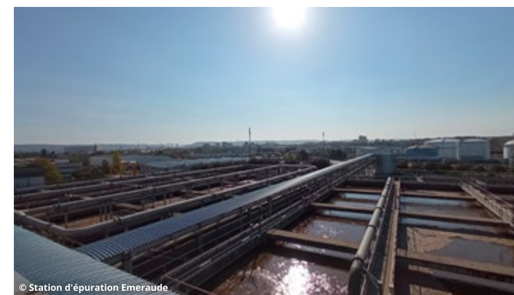
© Station d'épuration Emeraude
