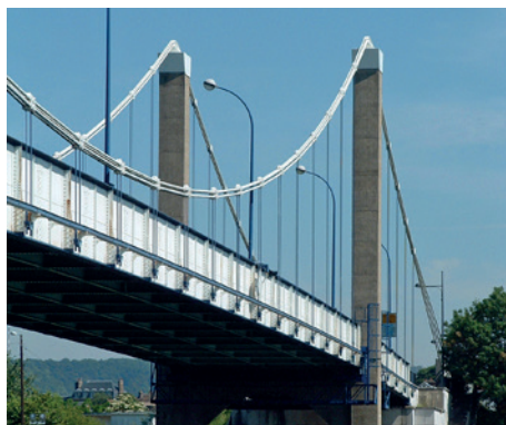
Pont Guynemer, Elbeuf © Mossot, Wikipedia Commons
